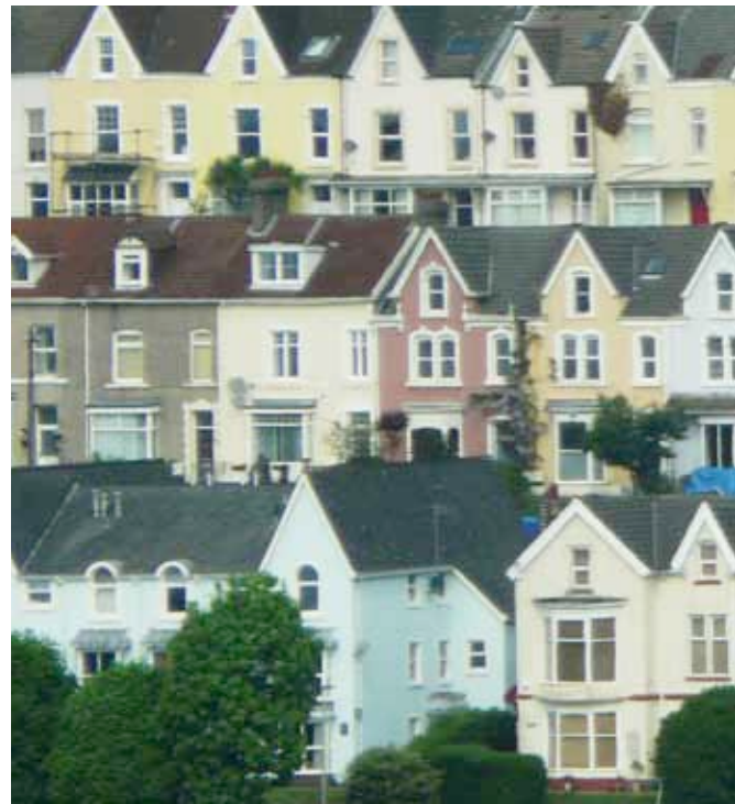
Houses in Swansea, Wales. Photo credit: Marie.
