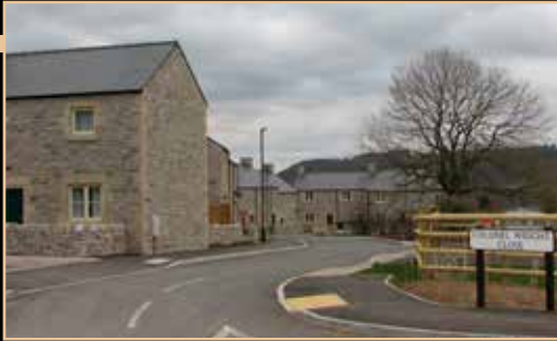
Colonel Wright Close, Bakewell submitted by Peak District National Park Authority Colonel Wright Close is a high quality development of 30 affordable local needs houses on an important gateway site in the Peak District National Park.
