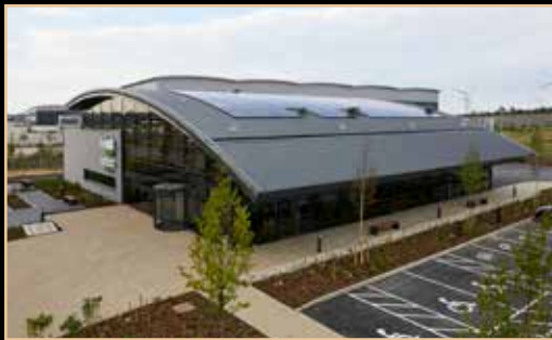
The Hub at DIRFT submitted by Lichfields and Prologis UK Ltd.
